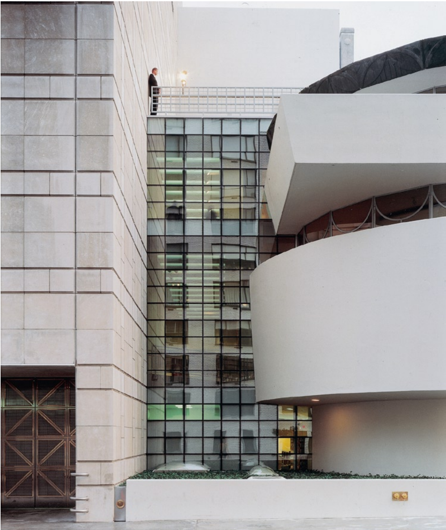
North facade showing infill glass wall
