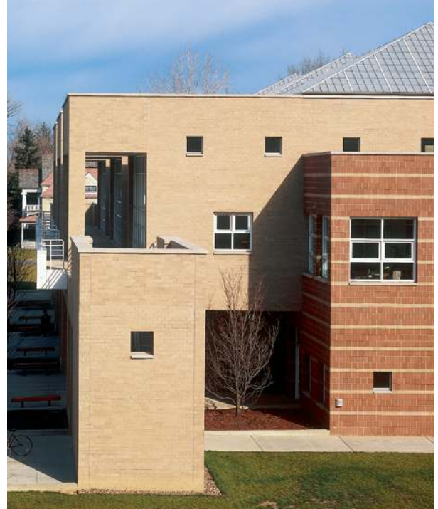
Corner of south facade
