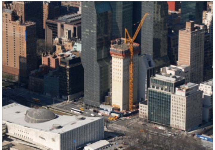
Aerial view of current construction progress
