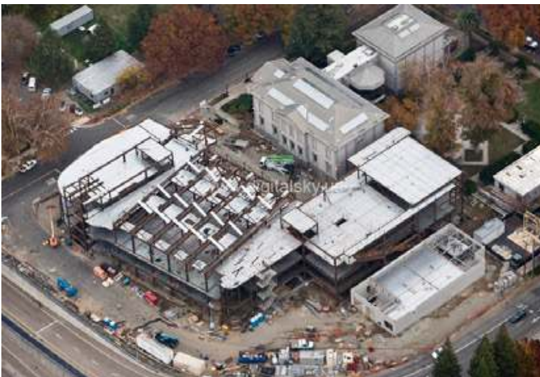
Aerial view of construction in progress
