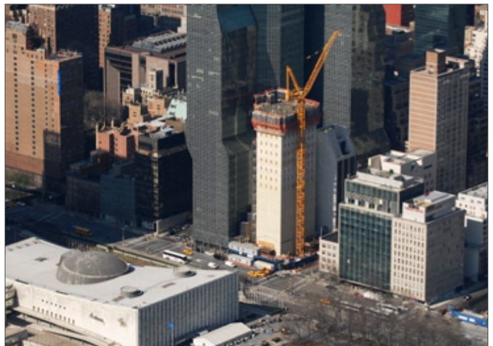
Aerial view of current construction progress
