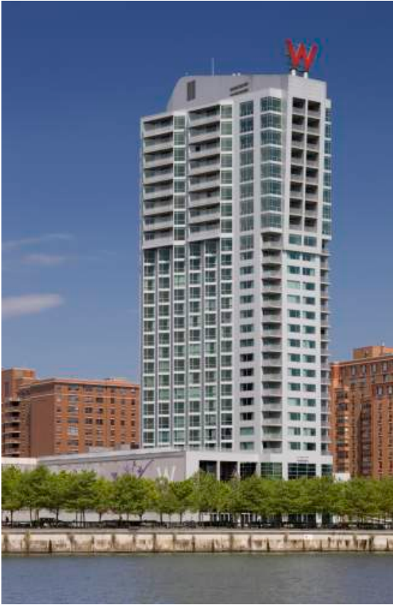
W Hotel Hoboken / photo and courtesy of Gwathmey Siegel Associate Architects
