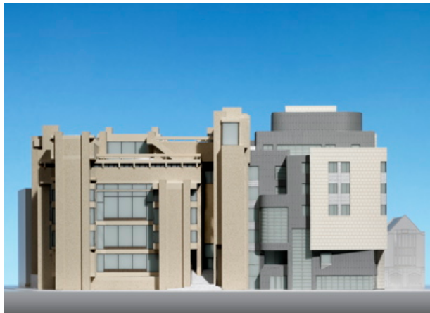
The Yale U. Art & Architecture Building, at left, is being renovated and an addition is being built, at right (Gwathmey Siegel image)
