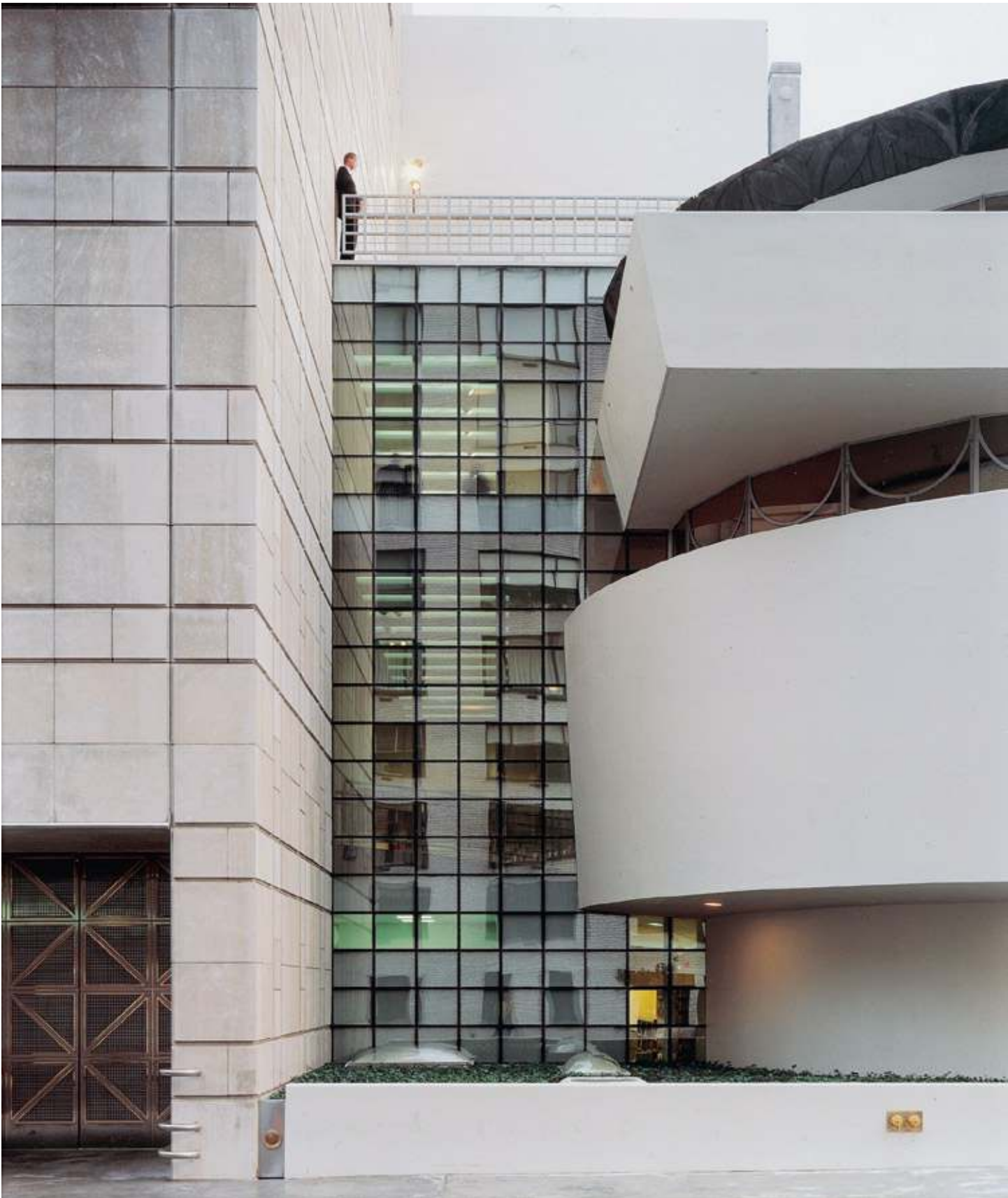
North facade showing infill glass wall
