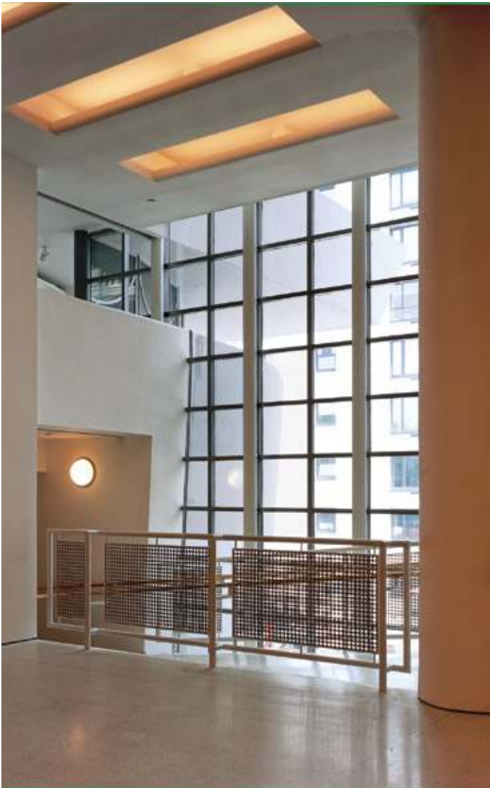
Infill glass curtain wall from second floor gallery
