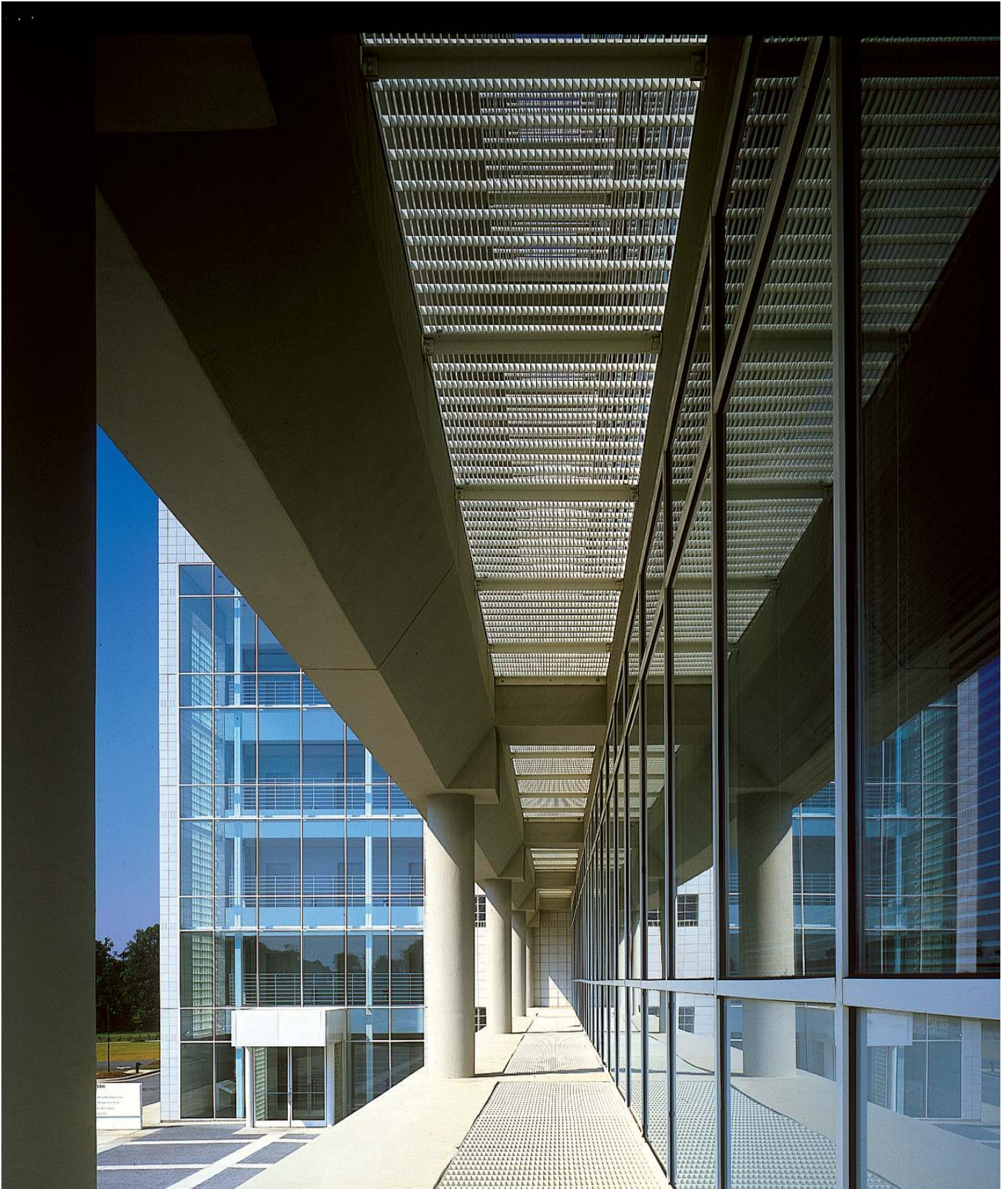
Detail of metal grating between brise-soleil and glass window wall
