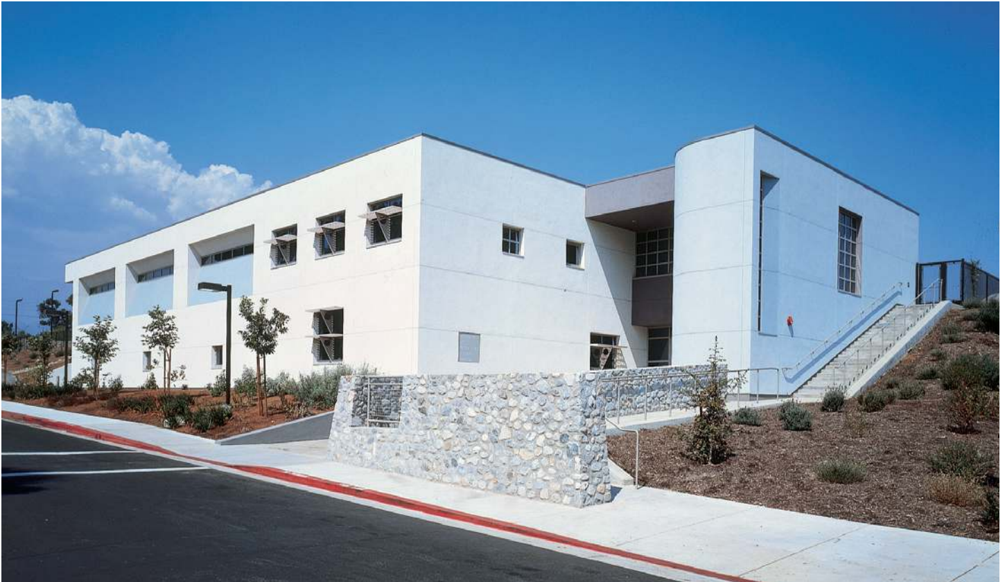
Gold Student Center, view of entry façade
