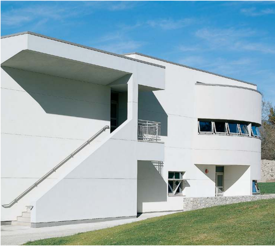
Campus green façade
