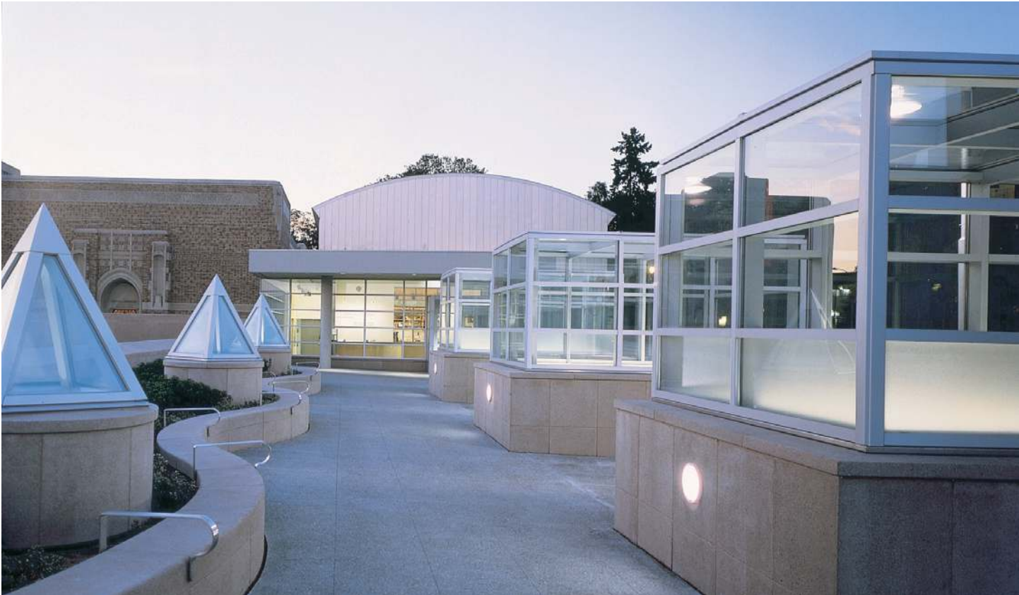
Plaza looking north toward new entry
