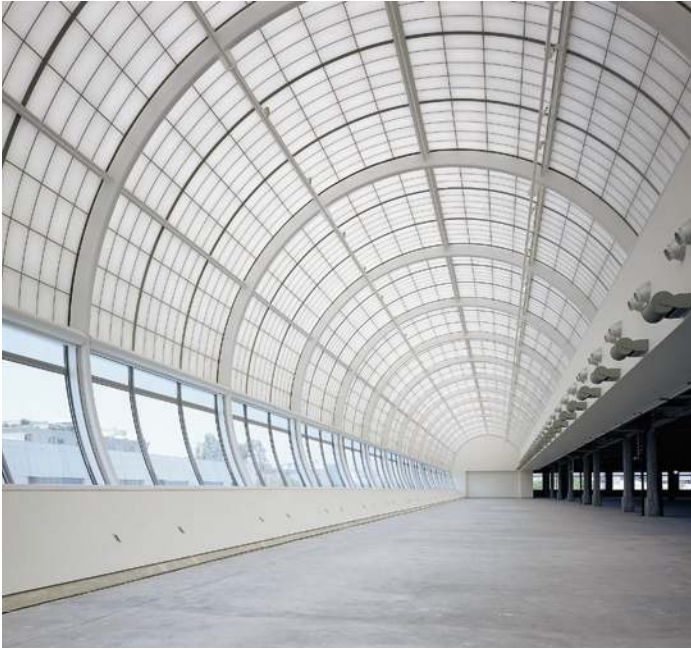
Interior view of translucent barrel-vault
