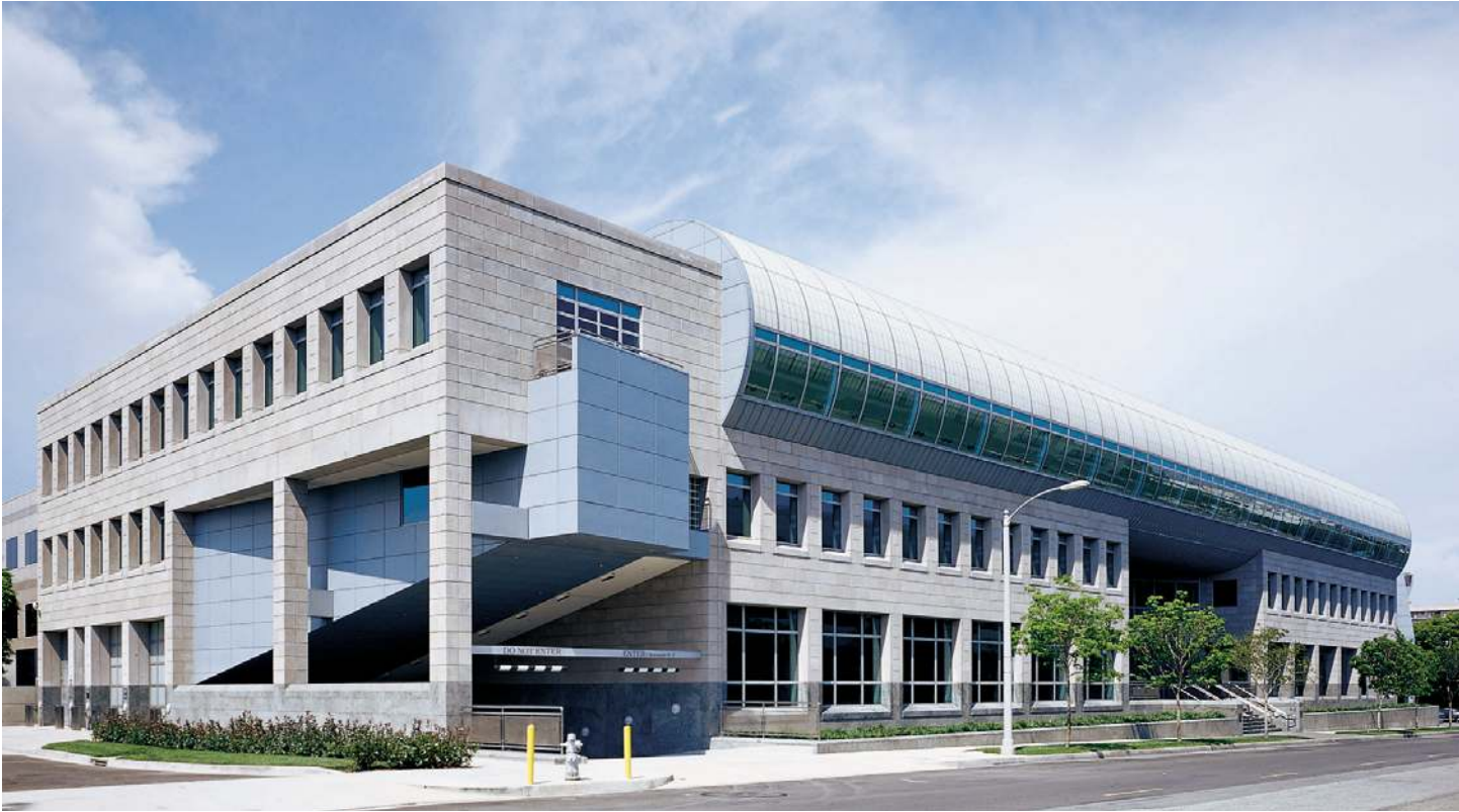
Exterior view from southwest with entrance to underground parking garage
