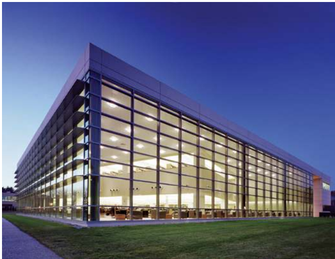
East elevation looking West
