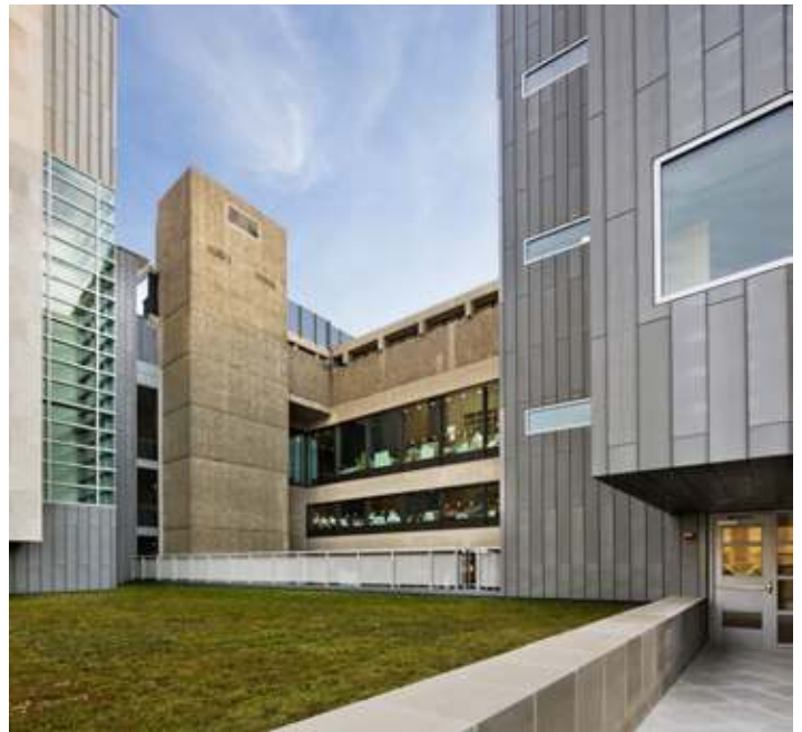
View of terrace and green roof
